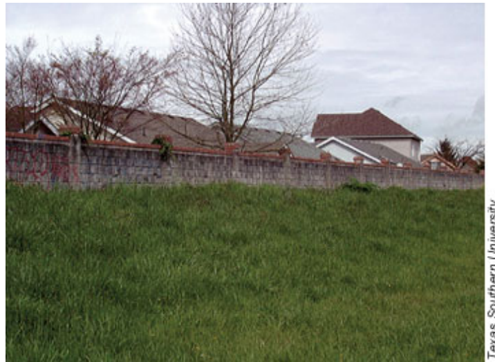
This privacy wall blocks residents' views of the highway and helps reduce traffic noise.
